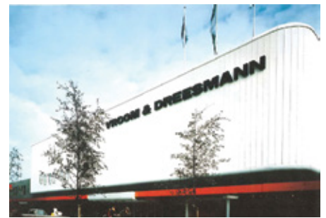
Shopping center (Netherlands)
