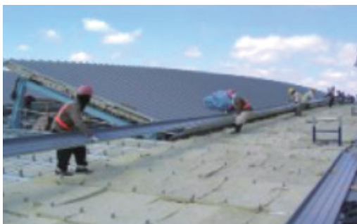
Simultaneous laying of roof panels
