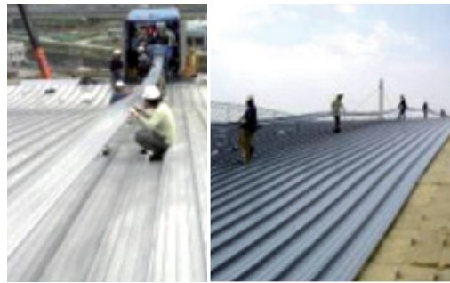
Metal sheet on-site molding
