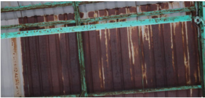
Original steel sheet roofing
