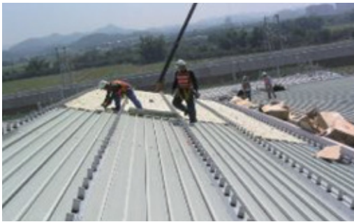
Bottom plate and insulation material laying, bracket installation
